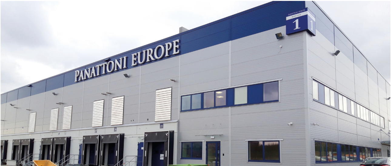
New modern and excellent located warehouse in Konotopa, close to Warsaw, dedicated to the Pharmaceutical Business.
