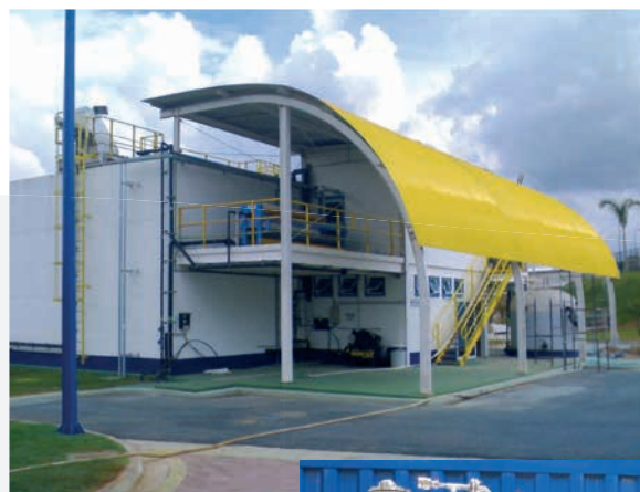
Modular plant system for the detoxification of wastewater at a pharmaceutical production site
