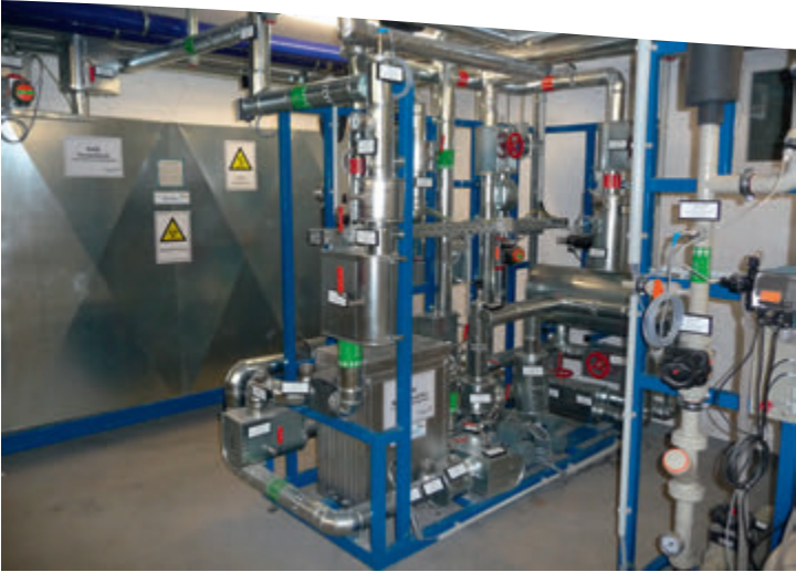
SteriFix E200 (200 l/h, 121°C, 20 min.) at Wacker Biotech showing the heat exchanger and the holding section – covered by insulation casing
