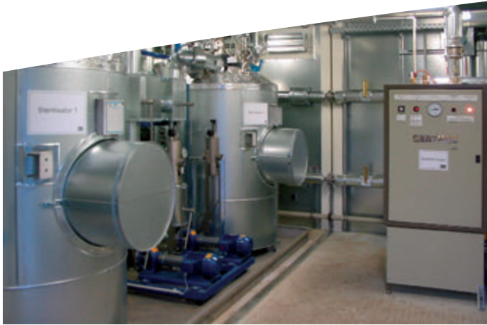
SteriFix C500/2S with steam generator (built as a modular plant in ISO shipping containers) at the State Office for Food Monitoring and Consumer Protection in Rostock, Germany
