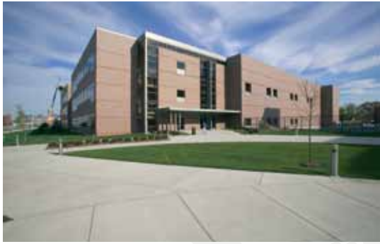
Biopharmaceutical API Facility (2005)
