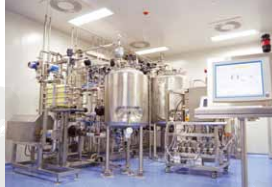
Bioengineering downstream skid
