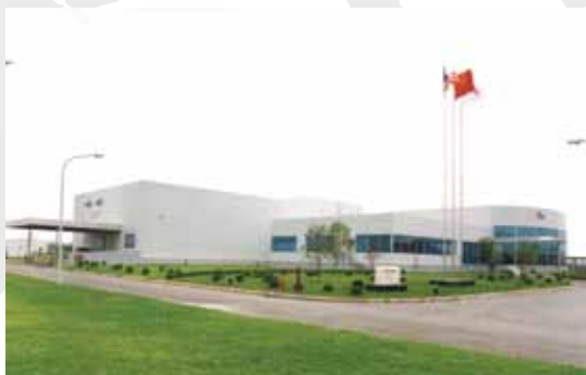
Solid Dosage Facility (1998+2000)
