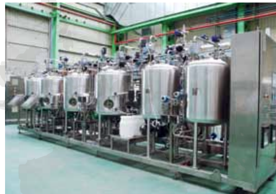
Other customized process skid
