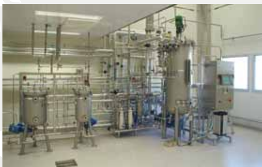
Biopharmaceutical API Facility (2002)
