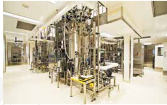
Biopharmaceutical API Facility (2007)
