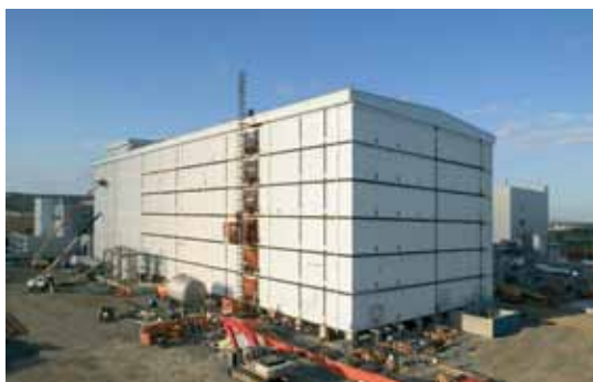
Biopharmaceutical API Facility (2004)
