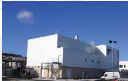
Biopharmaceutical API Facility (2005)
