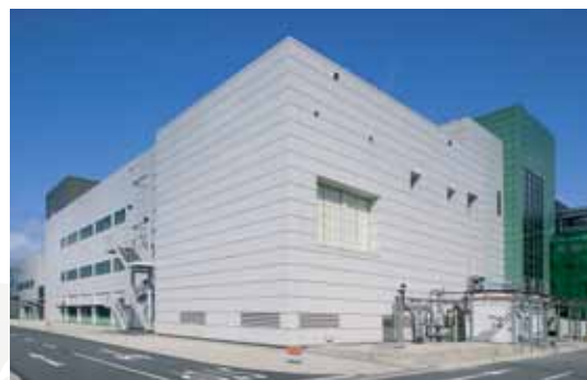
Solid Dosage Facility (2003)
