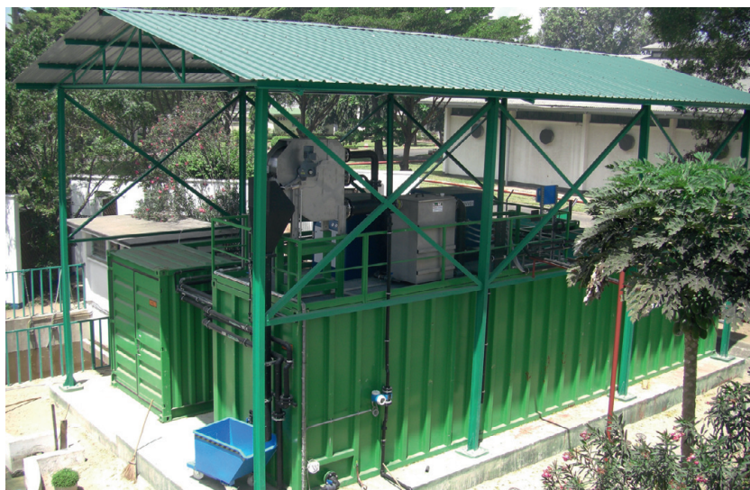
At a food manufacturer in Tanzania, process waters are treated physico-chemically and biologically for irrigation
